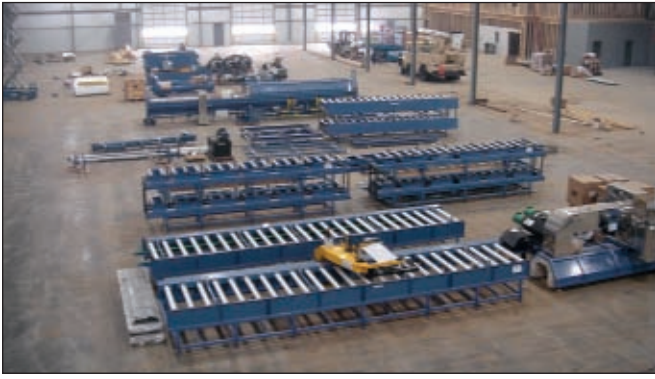
Figure 3. Installation of new equipment at Nappanee Window plant #4.
